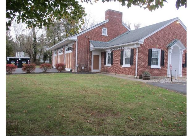
Rain gardens can be installed in the turfgrass area near the entrance of the building and near the parking lot to capture, treat, and infiltrate stormwater runoff from the roof and parking lot, respectively. Cisterns can be installed at the garage and main building to collect the runoff from the roof, which can be reused for washing vehicles or watering plants. A preliminary soil assessment suggests that the soils have suitable drainage characteristics for green infrastructure.
